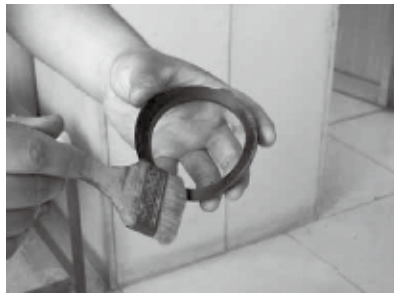
2. Spread lubricant on gasket ring.
