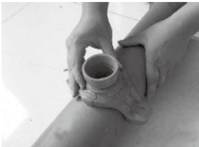
4. Install the Mechanical Tee in the hole.
